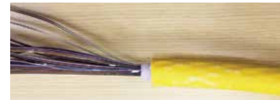
Stripping back cable
