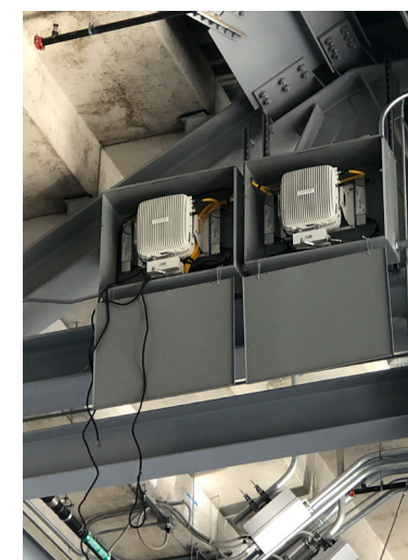
Clockwise from top: A MatSing antenna is lifted into place; DAS gear under the seating areas; looking down from a MatSing's location. Credit: ExteNet Systems
