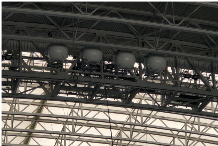
Clockwise from top left: A look inside the cavernous arena; scissor lifts help with installation; MatSing antennas painted to blend in. Credits: Top left, Todd Bergman, STR; other photos: ExteNet Systems.
