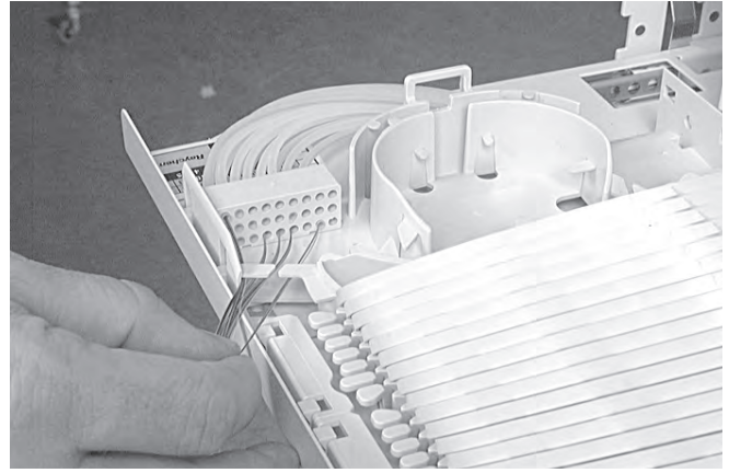
4.1.15 Pull the fibers at the other end of the tubes.
