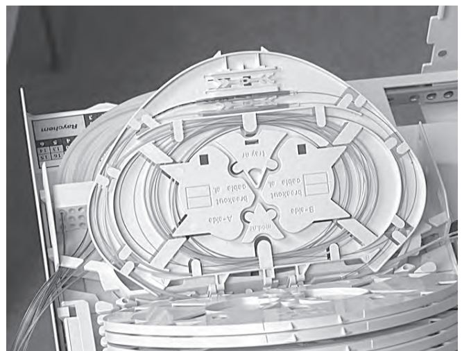
6.1.3 Store the fibers into the tray. Follow the exact routing as shown. Try to minimize the number of coils.
