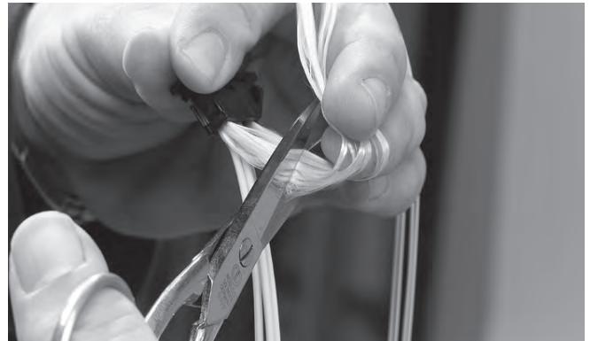
5.14 Pull the jacket and Kevlar at the same time to slide the inner part of the KTU into the outer part.
