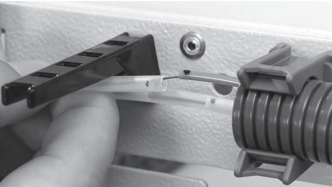
4.1.13 Select a loose tube and slide a 75mm long FOPT-CT over the transportation tube and loose tube or the transportation tube directly over the loose tube.
