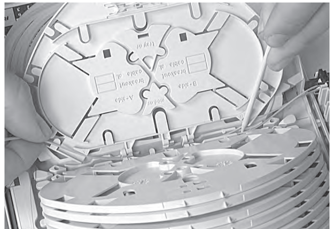
5.18 Guide the fibers into the corresponding groove. Make sure all fibers are positioned under the lips.
