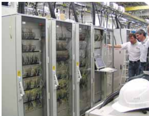
Above: Andrew engineers test the newly-installed ION-M system at an operator's dedicated BTS in the Allianz Arena, Munich. Left: A football enthusiast sends a photo to a friend.
