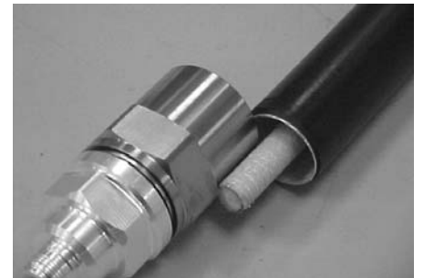
The cable end will look like this after Step 1. IMPORTANT: Confirm proper center conductor length by comparing to connector back nut barrel as shown.
