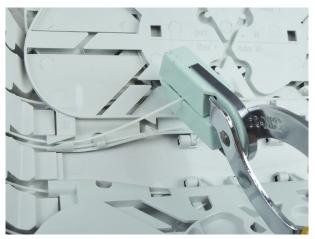
3.9 Strip the 900µm to 250µm with a proper tool
