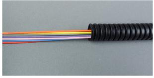
Feed the fiber through the flex tube 3.2
