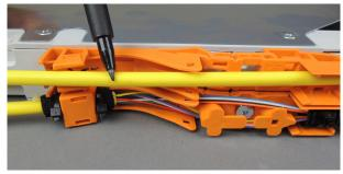
2.1.1 - mark the stripping point on the cable jacket - make sure you have at least 2 meters of cable left
