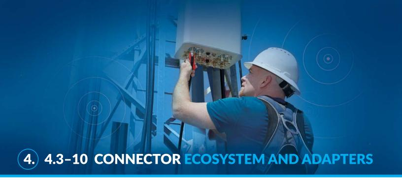
The additional inputs on modern antennas lead to a related challenge: the increasing density of connections at the tower top. Traditional DIN connectors are adequate when properly torqued, but installation errors are not uncommon and they can become a performance bottleneck. The likelihood of installation error only rises as more connections are packed into small spaces, which is why the new 4.3-10 connector standard is gaining such wide adoption.
