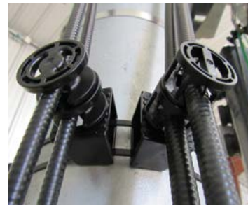
Hangers Installed with SA-1C
