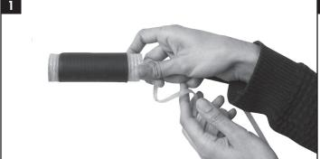
Hold shrink sleeve at a comfortable angle and pull the plastic tab until the front end of the plastic is removed and is even with the shrink sleeve (as is shown in 1b).
