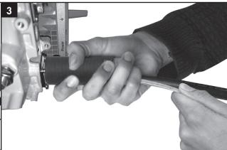
Slide the shrink sleeve forward over the connector assembly. Make sure the cold shrink is FLUSH against the connector cabinet. Hold the cold shrink in place over the connector to keep the sleeve from slipping. Your hand should be over the cold shrink and holding it in place against the cabinet as you start pulling the plastic tab away. Pull the plastic away until the cold shrink is fully deployed over the connector and cable (as shown in figure 4 on page 2).
