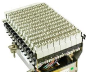
Figure 14: Pre-cabled cable head
