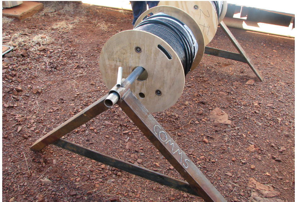
Pre-terminated sacrificial sheath cable is used to prevent termite damage
