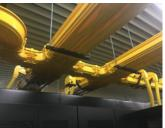
CommScope solutions employed in the deployment included indoor Cat 6 and Cat 6A (supporting wireless access points and video surveillance) unshielded copper cable; LazrSPEED 550 OM4 Bend-Insensitive multimode fiber; and TeraSPEED® OS2 singlemode Zero Water Peak indoor/outdoor common and outdoor dry armored cable solution.
