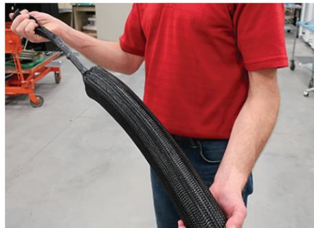
**5 Remove the pulling sock and protective wrap from the lead end of the cable, as follows (a-j below).**
