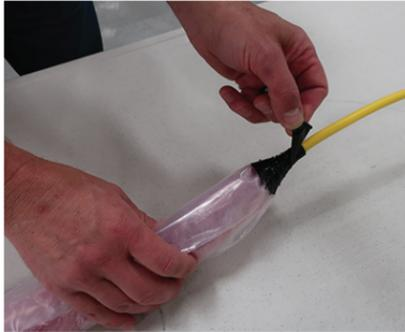
**6 Remove protective wrapping on second end of cable.**
