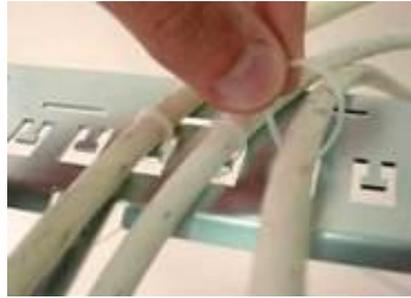
Use cable ties and fasten the cables. Do not fasten too tight to avoid cable deformation.
