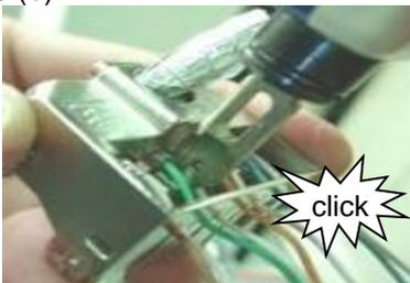
Alternatively to the Pistol Grip Tool, or for re-termination, terminate the wires using the Impact Tool on every wire.
