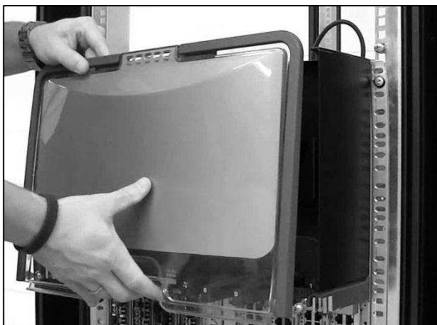
After all patch cords are installed, the plastic cover can be remounted.
