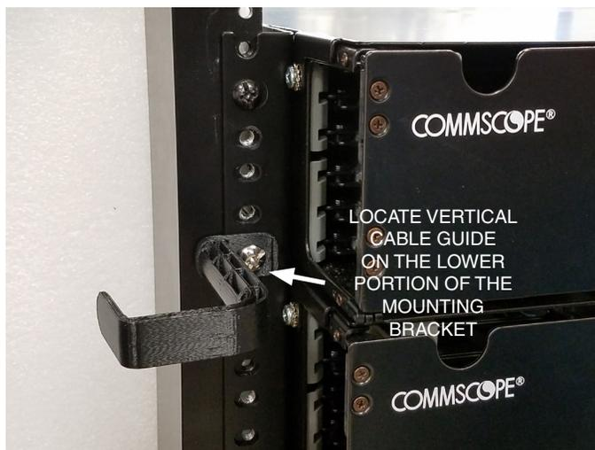
(3.) Connect Fiber Patch cords to module and run the cables out of chassis and over the accessory kit Vertical Cable Guide. Do this for both sides of the chassis.
