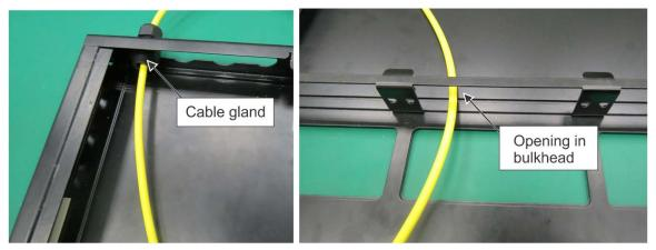
Figure 1. Install Incoming Fiber Cable
