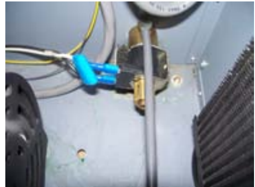
Figure 3 - Solenoid Valve With Rc Filter Wire Harness
