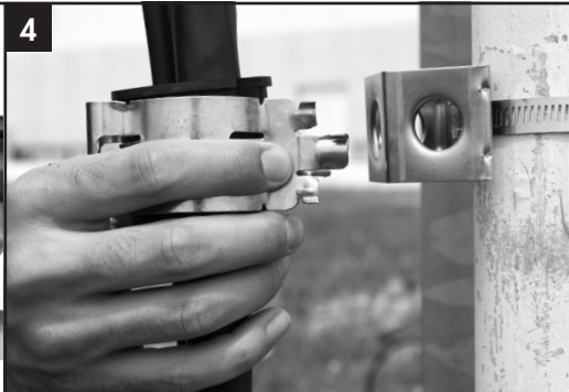
Insert SnapStak hanger into \frac{3}{4} " mounting hole adapter or cable ladder. SnapStak hangers can be stacked 2 high maximum.
