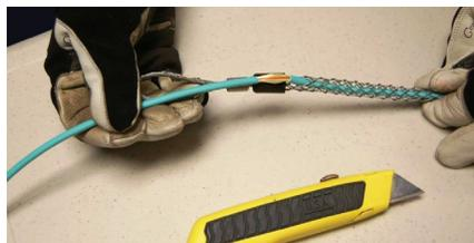
4. Twist the yarn into a manageable bunch and tie it securely to the pulling eye of the mesh grip.
