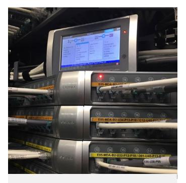
The imVision® AIM platform delivers a holistic view of the network connectivity in real time. Intelligent software, network controllers and accessories allow network managers to locate and identify equipment and ports and track all network changes. It also guards against unauthorized physical intrusion and automatically documents all changes. team completed the initial design, it focused on finding the right cabling partner.
