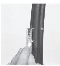
10 Place a second mark on the cables 30mm below the first mark (for PEDCAP-R-3, R-4S and R-4L only).
