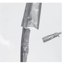
5 Temporarily position the Aluminium bag over the joint to protect joint and conductors from damage (flame protection). Do not tape. Flame brush the abraded area of each added cable for 10 seconds.
