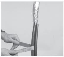
7 Using the kitted abrasive strip, abrade the cables circumferentially over a distance of about 150 mm for PEDCAP-R-3 and 250 mm for PEDCAP-R-2 and PEDCAP-R-4S/4L, from the sheath cut.
