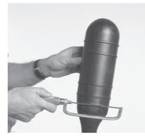
1 Make a ring cut with a hacksaw at the top of the transition area, without damaging the installed joint and conductors. Remove the dome of the PEDCAP.
