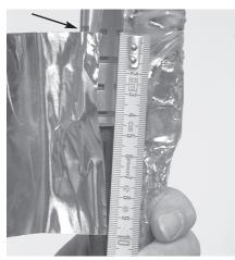
7 Apply one layer of aluminium cable foil around the ADDED cable. Start at 30 mm, or the 3rd SCOP slot from the end, away from the completed joint, in the direction of the cables. Smooth the foil with a blunt tool.
