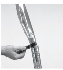
15 **For PEDCAP-R-3 and R-4S/4L** form the cables into a tight bundle (secure the silicagel to the joint). Slide the aluminium bag completely over it and secure with PVC or heat resistant tape. Do not tape more than 20 mm, or the second slot, onto the SCOP.
