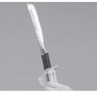
6 Using the kitted cleaning tissues, clean the cables for a distance of about 300 mm starting from the cable sheath cut.
