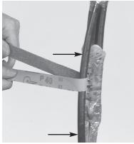
4 Clean the added cable, using the kitted cleaning tissues. Using the kitted abrasive strip, abrade the added cable in the area of the SCOP (installed on the other cables). **Remove temporarily installed local approved tape from existing SCOP**.
