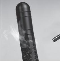
16 Install the PEDCAP over the joint and start shrinking the PEDCAP from where the Thermo-indicating (TI) paint is applied on the body and move towards the end of the closure, converting all TI paint to black.
