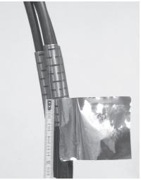
12 Apply one layer of aluminium cable foil around each cable. Start at the 3rd SCOP slot from the end, away from the completed joint, in the direction of the cables. Smooth the foils with a blunt tool.
