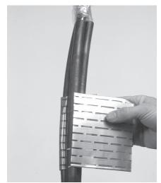
11 Install one SCOP on EACH cable, positioning them between the LOWEST mark and the completed joint. Apply SCOP tightly around each cable in the direction as shown on the backing paper, not more than two layers. **Note: for cables with diameter less then 8mm: the SCOP-200 may be cut longitudinally in halves following the cable** drawing on the backing paper. Apply one half to each small cable in the direction as shown on the backing paper.
