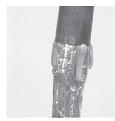
18 Leave the closure undisturbed for a minimum of 30 minutes.
