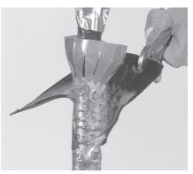
3 Remove the pre-heated sleeve with a pair of pliers. **Note**: when removing a PEDCAP-R-4S/4L, if present, remove any inner cardboard liner. Apply additional heat to facilitate removal if required. Remove the taped aluminium bag completely.
