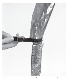
11 **For PEDCAP-R-3 and PEDCAP-R-4S/4L** form the cables into a tight bundle (secure the silicagel to the joint). Slide the aluminium bag completely over it and secure with PVC or heat resistant tape. Do not tape more than 20 mm, or the second
