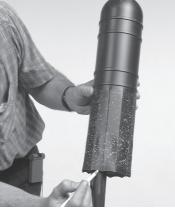
9 Position the PEDCAP completely over the joint. Mark the cables at the bottom of the PEDCAP and remove the PEDCAP and aluminium bag.
