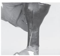
2 Heat the recovered sleeve area. Make a longitudinal cut in the pre-heated sleeve area without damaging cables or joint.
