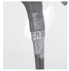
17 Continue heating with a soft flame until the adhesive flows at the end of the PEDCAP and **between ALL the cables**.
