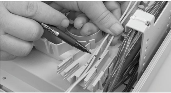
3.6 Route the loose tube towards the tube holder and strip.
