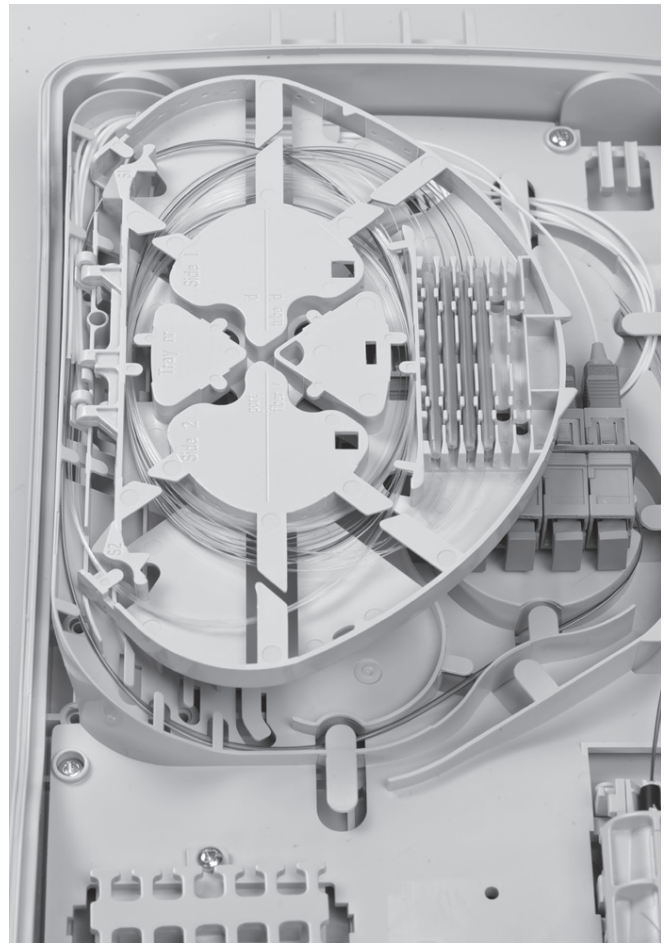
4.8 Splice the fibers from the feeder cable to the pigtailed and store the overlength into the tray.
