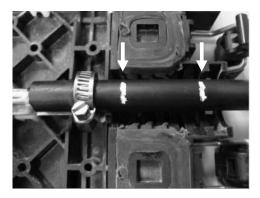
5.8 Install the cut rings on the cable.
