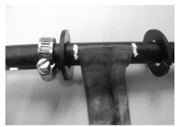
5.10 Diameter of wraped gel strip should be one circle higher than ring. Cut the gel tape at the direction of the bending of cable bracket which can ensure the sealing by keeping the gel strip opening under the cable.
