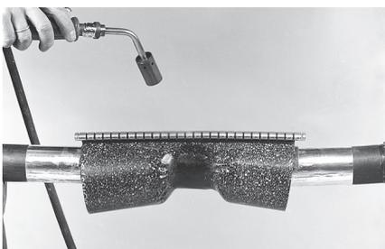
**16** Center the sleeve and start recovering it in the middle on the opposite side of channel. Heat until the paint changes colour from green colour to black.
