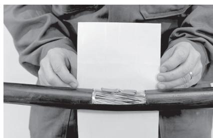
**5** Install the liner around the cable opening such that the middle of the liner matches the middle of the splice. Wrap tightly around the cable and smooth alu-liner; cut it to size such that there is a 40 mm overlap.
