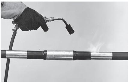
**13** Flame brush the entire cable surface to be covered by sleeve for about 10 seconds on each side of the splice. For lead cables preheat the lead up to  $\pm 60^{\circ}\text{C}$  (hot to the touch).
