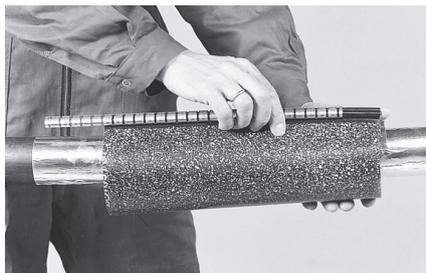
**14** Install the heat-shrinkable wraparound sleeve around the splice. Pull the channel over the rails.
