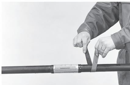
**8** Abrade the cleaned area of the cable circumferentially. Remove abrasion dust with a clean, dry cloth.
