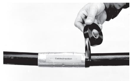
**6** Tape, the liner down onto the cable on both ends. Tape maximum 5 mm on the cable to avoid shortening of the bondlength.
