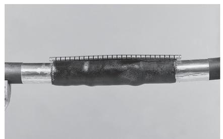
**18** Repeat step 17 at the other end of the sleeve. Allow the sleeve to cool down to ambient temperature before any handling and repressurizing the cable.
