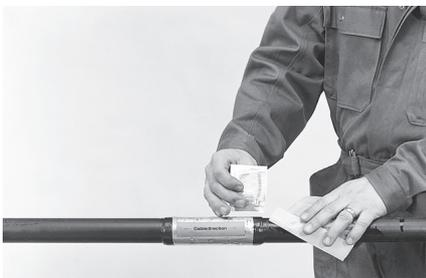
**7** Clean the entire circumference of the cable jacket over a length of 200 mm on each side of the liner. Use a cleaning tissue supplied in the kit.
