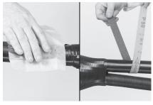
**9** Remove solvent impregnated tissue from its package and clean all cables for a distance of 20 cm. Abrade all the cables circumferentially over the same length.
