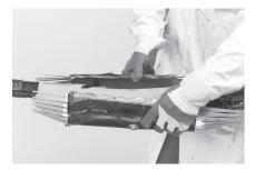
**9** Remove the canister and rework the splice.
