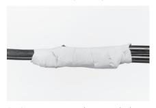
**5** Construct joint according to standard procedure and wrap joint with insulating material (not included in standard kit).
