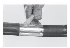
**12** Smooth the aluminium tape with a blunt tool to smooth sharp edges.
