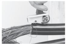
**2** In order to install the shield continuity assembly, cut the cable jacket over a length of 25 mm and a width of 10 mm. Put cotton tape (not included in the standard kit) underneath the cable jacket strip.
