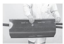
10 Center the sleeve over the canister by placing the metal ring in the sleeve over the valve in the canister. Mark ends of sleeve on cable Jacket.
