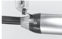
**8** Using PVC-tape (not included in standard kit), tape the crowns, starting from the canister body, down to the cable.
