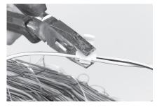
**4** For joints with more cables at one end install the branch continuity wire assembly, using a crimp connector.
