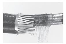
**6** Remove tape on the crowns of the canister
