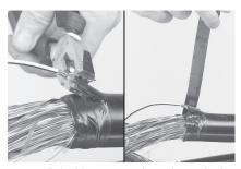
**3** Install shield continuity clip with standard pair of pliers and wrap the entire shield continuity connector with PVC tape (not included in the kit).
