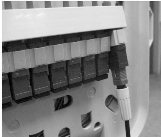
10.6 Remove the drop cable dummy rods
