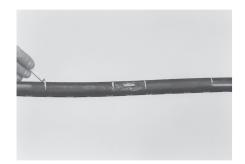
4 Measure 12,5 cm out from the repair area on each side and place mark on the cable sheath.
