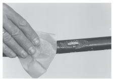
$2\,$  Clean and degrease the cable sheath for a distance of sleeve length + 25 cm.
