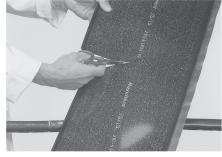
8 Cut the CWST to length with cutter, knife or with scissors. The cut must be perpendicular to the axis of the sleeve.
