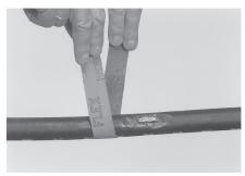
3 Abrade the cable sheath circumferentially over the same length. Use local practice to abrade lead sheathed cable.
