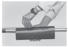
12 Remove the release foil from the inner side of the wraparound, assemble the wraparound sleeve over the cable and slide on the metal channel. If two channels are needed press the retention clip over the rail at the center.
