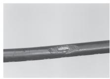
1 Select the proper size of cable repair sleeve. The sleeve length selection is defined by damaged area length + 25 cm.
