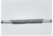
17 Repeat operation from the center to the other end of the cable repair sleeve. The visual control for proper installation should be done now:
