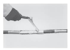
3 Remove the aluminium flap of the sleeve with pair of pliers. If necessary reheat the aluminium flap gently.
