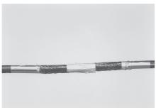
4 When the CWST is removed, the remaining adhesive may be left on. However, protect the adhesive from contamination (grease, mud, dust, etc...) with cotton tape or similar.
