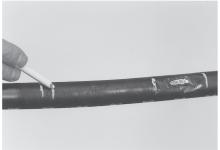
5 Make second mark at 1 cm from the first mark towards the repair area. (Not applicable for lead sheathed cable).
