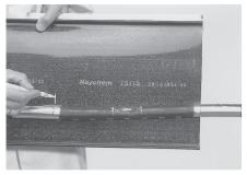
7 Align one end of the CWST sleeve 1 cm over the aluminium tape. At the opposite end, mark the sleeve length at 1 cm further the aluminum tape.
