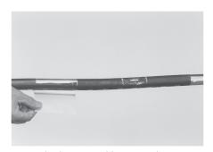
6 Apply aluminium cable tape on the PE-cable sheath away from the repair area starting from the inner mark. (Not applicable for lead jacketed cable).
