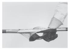
2 Heat the sleeve uniformly till it opens at the channel area. Grip the edges of the sleeve with pair of pliers and peel the CWST off the cable.
