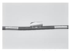
10 Important! In case the cable sheath is damaged down to the aluminium layer of the cable sheath, protect the repair area with an aluminium tape or similar. This avoids the hot melt adhesive flowing down to the cable wrap.
