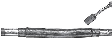
**22.** After complete installation of the second tube give a post heating of 15 seconds around the middle of the tube.
