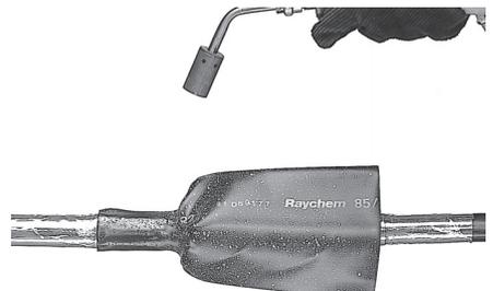
**15.** Start heating at one end of the tube. Shrink the tube end over a distance of approximately 70 mm. Apply heat until all the temperature indicating paint has changed colour from green to black. Move flame continually to avoid local overheating.
