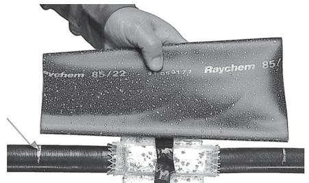
**12.** Centre the shortest tubular sleeve over the adhesive bags and mark the tube ends on the cable.
