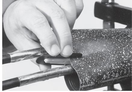
6.6 Shrink the oval cable seal on the FOSC-base side with the recommended hot air gun device with reflector. Shrink sleeve until the green thermo-indicating paint is converted to black. (Make sure the hot-air temperature is at least 350°C). (If a FACC-HEAT-GUN-220V is used, set position on scale 10).
