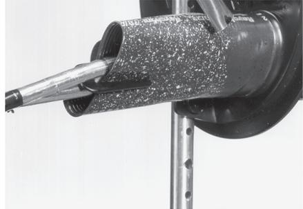
6.7 Shrink down the end of the sleeve on the cable side. Heat until the sleeve shrinks down on the cables and take care that the green thermo-indicating paint is converted to black. Postheat the clip on both sides till the adhesive shows a proper flow on the clip between the two cables.
