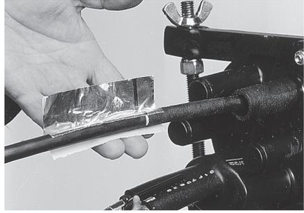
11.10 Slide the cable seal over the port. Shrink the cable sleeve on the base side with the recommended hot air gun. Use the reflector to ensure heat distribution around the outlet. Shrink sleeve until the green thermo-indicating paint is converted to black.
