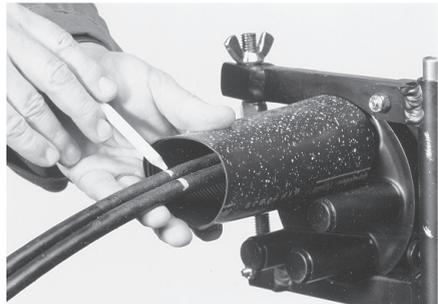
6.4 Match the blue line of the aluminium cable protection foil with the marks on the cables. Wrap aluminium cable protection foil around cable.
