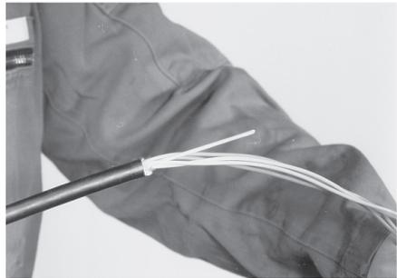
5.2 If a shield continuity is required, cut cable sheath axially for 25 mm from cable ring cut. Crimp shield clip on cable sheath with pair of pliers. Protect the clip with self adhering tape.
