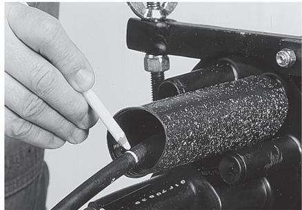
11.9 Match the blue line of the aluminium cable protection foil with the marks on the cables. Wrap the aluminium cable protection foil around cable.
