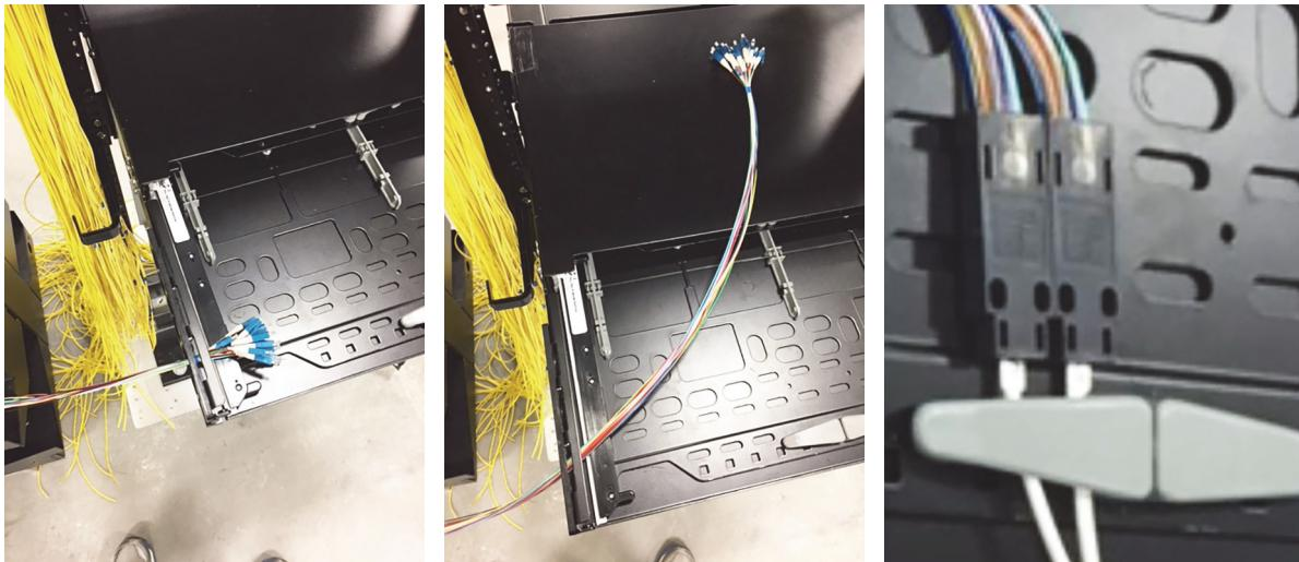
4. Gently start laying the fibers down on the tray (easier with two people) wrapping it around in about a 4 inch circle until you can snap the fiber adapters into place.
