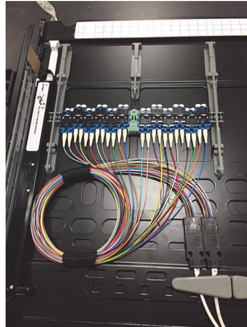
6. Make sure no fibers are sticking up in the air, stretched, or pinched. Repeat procedure for other half of the tray. When finished with both sides, add a piece of yellow tape supplied over the top of the fanouts.
