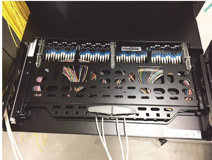
8. When all trays in the chassis are completely populated and pushed back into the chassis, then you can secure the tails, there should be about 25-30 inches of slack of the 3mm cable in the back of the panel. Stick down the cable tie just inside the entry port at a 45 degree angle. Wrap the cables with felt tape and secure cables with two zip ties.
