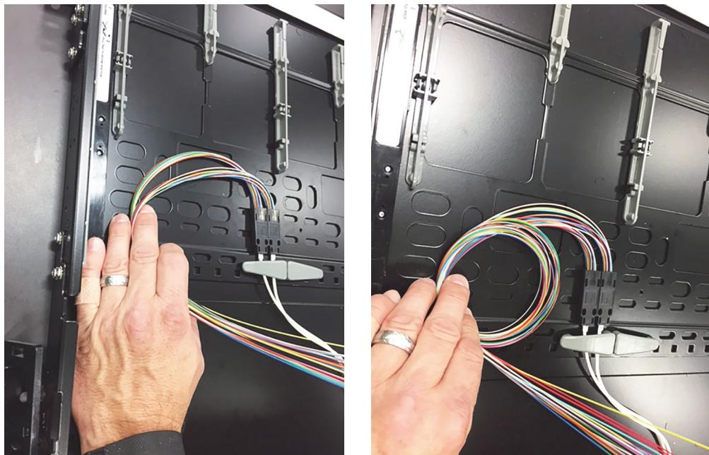
5. While holding it all, gently wrap the Velcro around the fibers in two places to hold the fibers securely.
