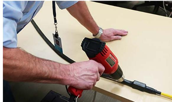
15. When the assembly has fully cooled, remove the foil tape from the mesh sleeve.
