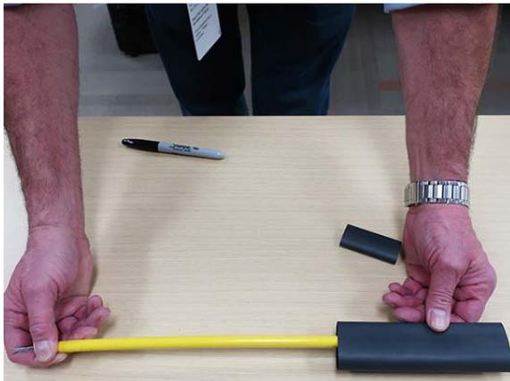
3. Slide one of the two pieces of 2.5-inch (6.4 cm) heat shrink tubing over the cable stub end.
