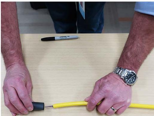
4. Slide the 2.5-inch (6.4 cm) heat shrink tubing up the cable and out of the way.
