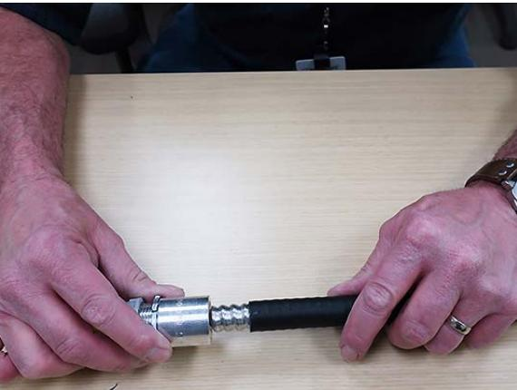
9. Slide the heat shrink tubing over the rear of the armor fitting until it reaches the flange at the end of the armor.
