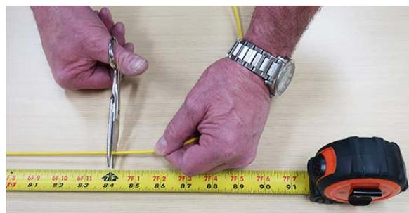
**Note:** The furcation tubing length will be determined by the final fanout kit location within the rack or cabinet and the desired length of service loop between the fanout and the cable entry point into the fiber shelf PLUS 33 inches (84 cm) of length within the fiber shelf. The typical minimum furcation tubing length is 72 inches (183 cm), typical maximum length is 93 (236 cm) inches.
