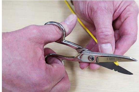
6. If ribbon fibers are grouped by binder yarn, undo one group at a time as ribbon fibers are inserted into the furcation tubes. If present, trim binder yarn to expose 1/2 inch (13 mm) or less.
