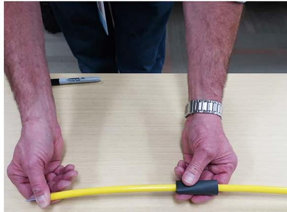
5. Measure and mark the cable sheath at 96 inches (244 cm) from the stub end of the cable.
