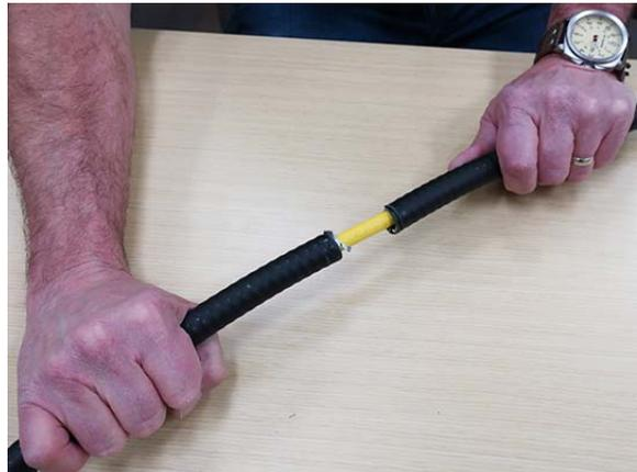
4. Slide the heat shrink tubing included in the armor kit over the end of the cable.
