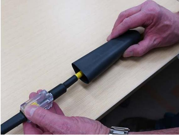
13. Center the 6-inch (15.2 cm) heat shrink tubing between the fused edges of the cable and mesh sleeve.
