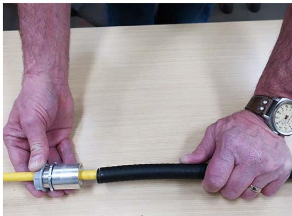
7. Trim back the armor jacket about 1 inch (2.5 cm) to prepare a place for the armor fitting to be threaded onto the interlocking steel armor.
