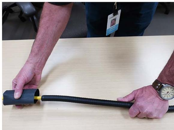
5. Slide the heat shrink tubing up past the cable armor and out of the way.
