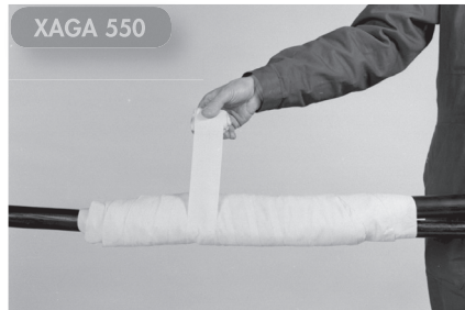
8A Wrap joint with tape (paper insulating tape, cotton tape or equivalent - not included in standard kit). Taped length should not exceed the length inside the liner/metal canister.
