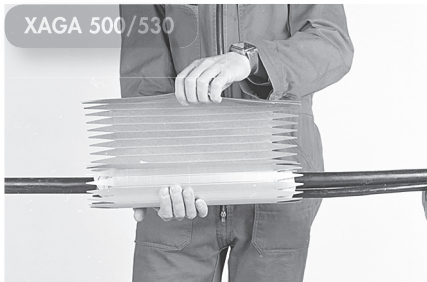
7 Before installation of the liner, preshape the liner cylindrically by rolling. Wrap the liner tightly around the splice bundle and secure with tape.
