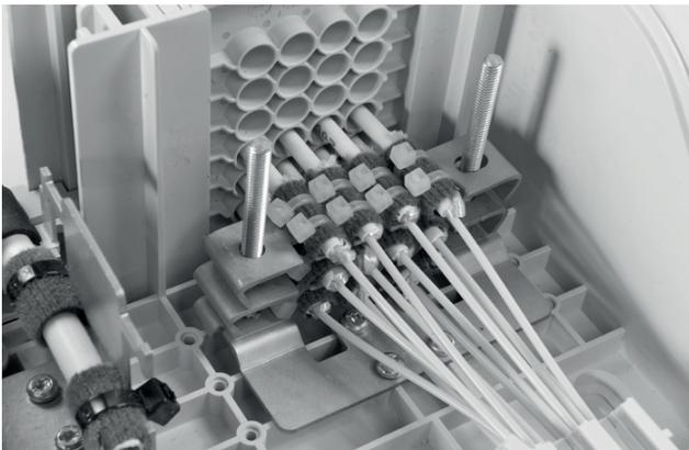
3.1 Install the drop cables into the ports.
