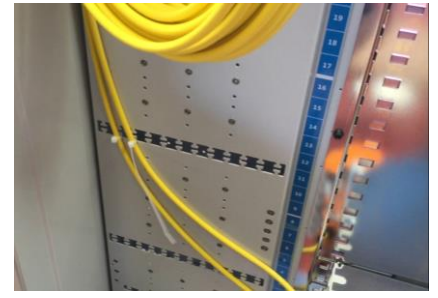
4.1.6 Fix the cable on the side duct Using a cable tie
