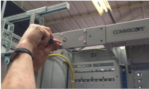
4.1.7 If the cable is not initially threaded through the top of the rack, a removable panel allows cable routing after the shelf is installed.
