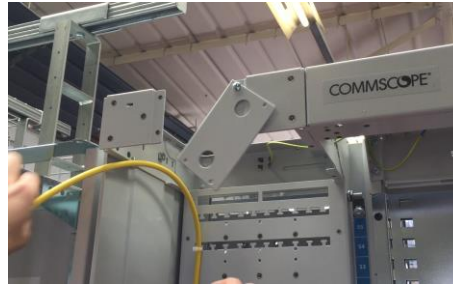
4.1.8 Unscrew the panel bolts as shown, and pass the cable through.
