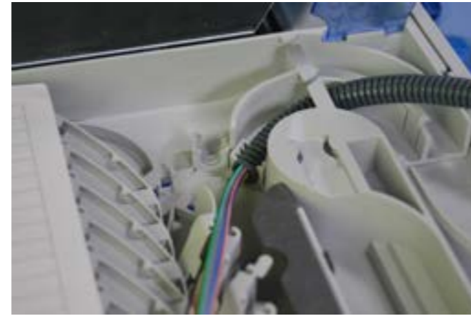
6.6. Guide the flex and the 900 µm fibers to the splice tray. Fix the flex tubes in the flex tube holder.
