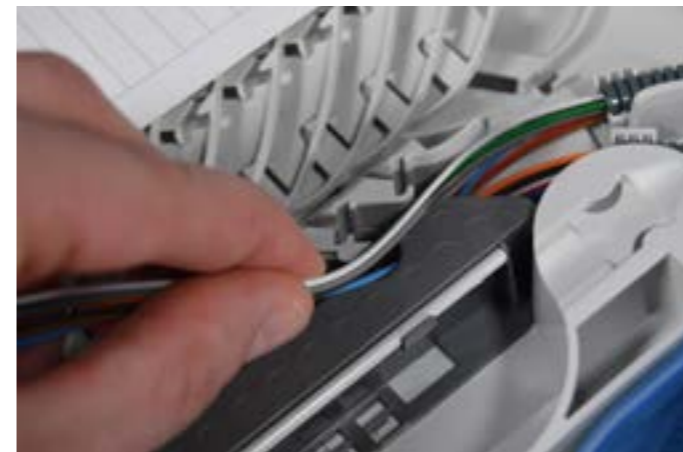
6.8. Route the fibers throughout the groove plate to the dedicated splice trays.
