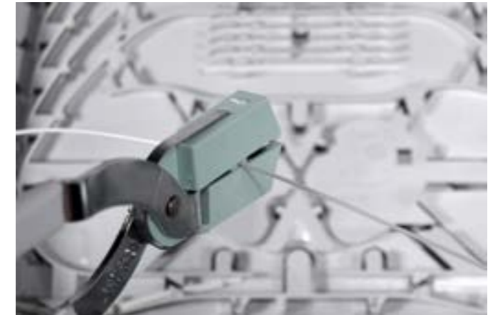
6.10. Strip the 900 µm to 250 µm with a proper tool.
