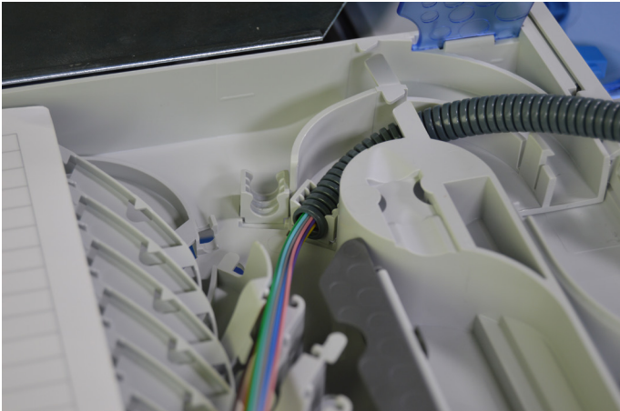
6.6. Open the lids. Guide the flex and the 900 µm fibers to the splice tray. Fix the flex tube in the flex clip.
