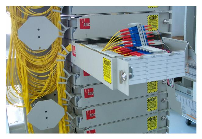
13. Re-connect the connectors. Figure 10 shows the adapter pack with the connectors installed.
