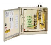
IFDH 3000 Indoor Fiber Distribution Hub, 144F, SC/APC, riser ribbon stub,100ft, spliced input, 24FF
