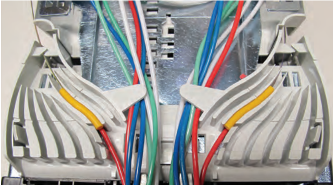
11.3.8 Press the piece of orange tubing in the groove on top of the tube/subunit. Note: place the end of the orange tube/subunit at the start of the groove. This makes it easier to remove the orange tubing.
