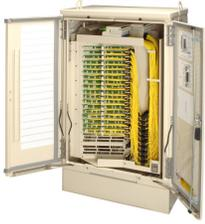
Standard FDH3000, 576F loaded pole (bottom entry) mounted cabinet, SC/APC, PNP splitter capable, OSP Dry Dielectric Flat Ribbon Cable, 100 ft stubs, using 2x288F distribution cable assembly and 1x96F feeder, Build America Buy America (BABA)\* Coming soon
