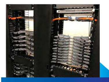
"The infrastructure used in the data center, combining a 6A structured cabling system and OM4 multimode optical fiber, was designed for high performance. Moving the data center was included in the project. We have considerable experience in this type of work in large industries and carried out careful planning to ensure the move was seamless and on time."
