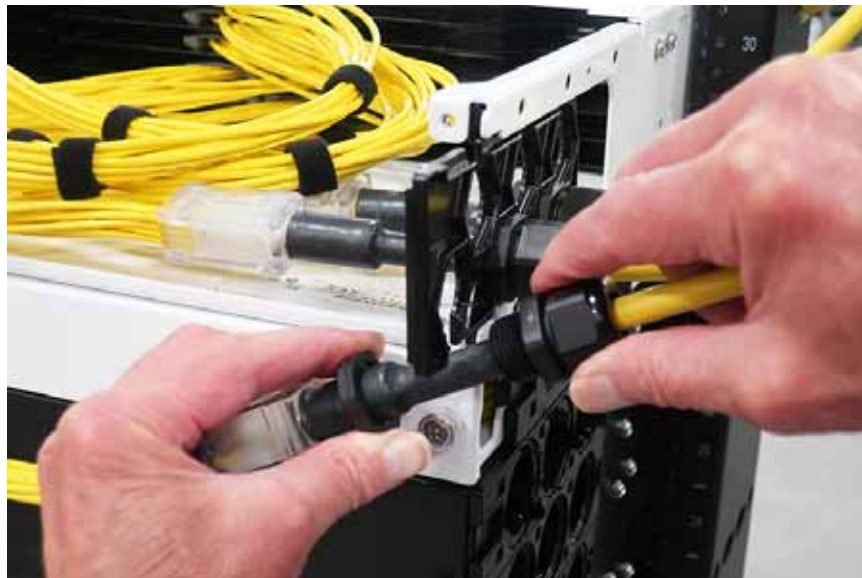
Figure 20. Inserting Cable Into Knockout Opening
