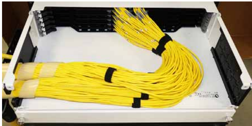
Figure 25. Cable Routing from One Side (Overhead View)
