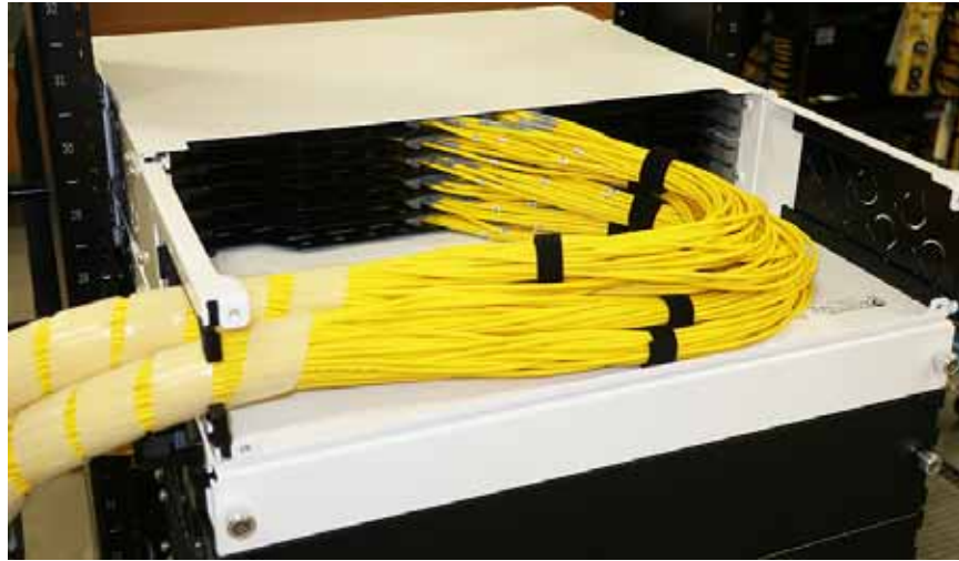
Figure 24. Cable Routing from One Side (Side View)
