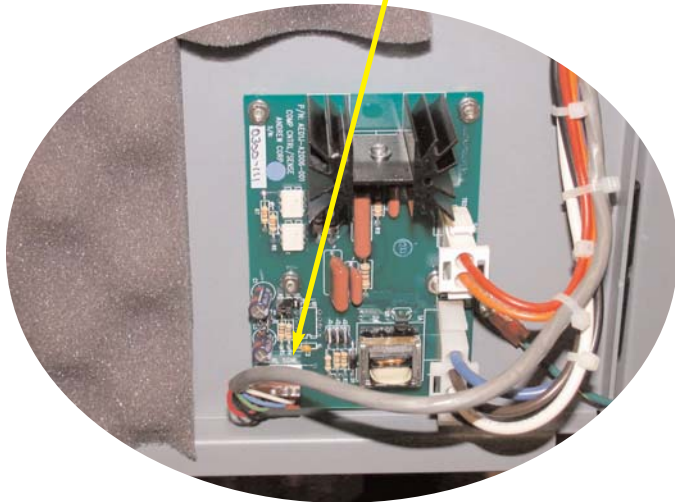
Slave unit cable connection (for reference, factory installed).
